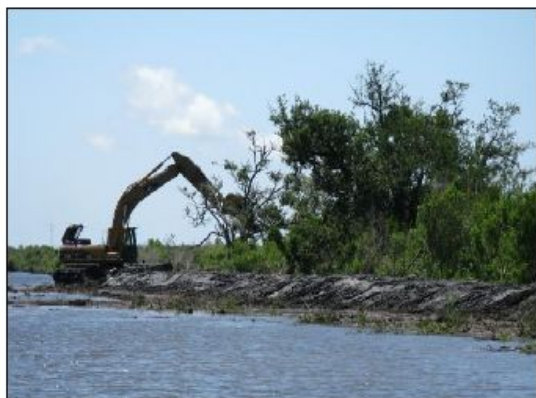
Bayou Dupont, LA Coastal Restoration
