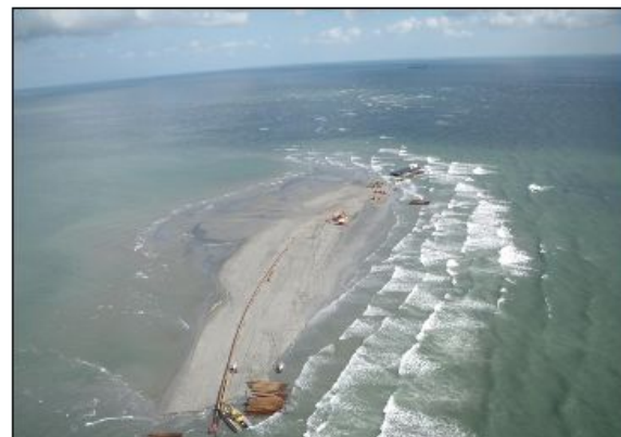
Berm construction off Louisiana coast
