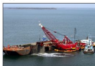
Dredge GL 55 at Upper Chesapeake
