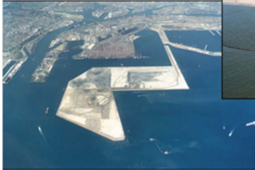
Capital Deepening ports, land reclamation, and excavation of underwater trenches
