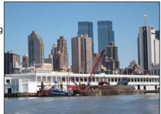
Dredge 54 at NYCT Berth
