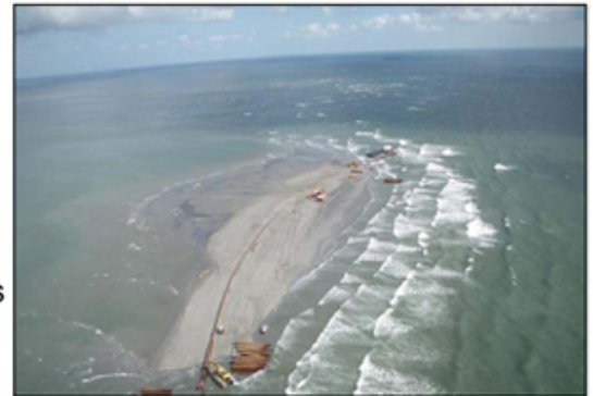
Berm construction off Louisiana coast
