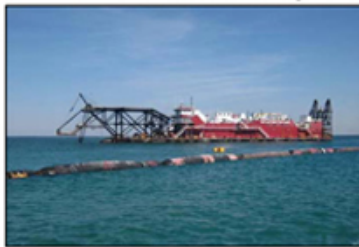
Dredge Texas at Boca Raton
