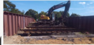
EXPANDING DEMOLITION BUSINESS
