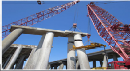
I-10 Bridge Project in Louisiana
