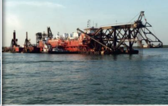
Cutter Suction Dredge Texas excavates material in Miami Harbor
